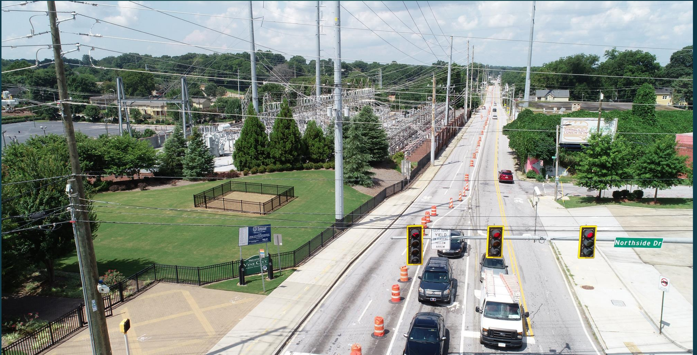
Boone Bridge - Before
