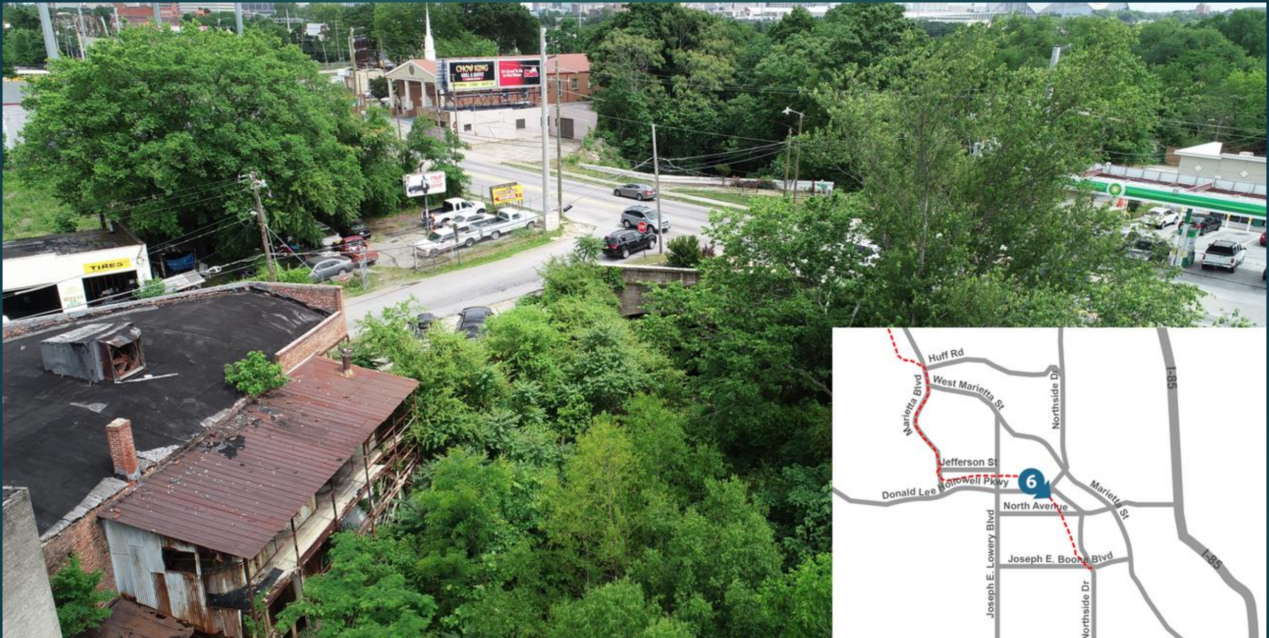
Donald Lee Hollowell Tunnel - Before
