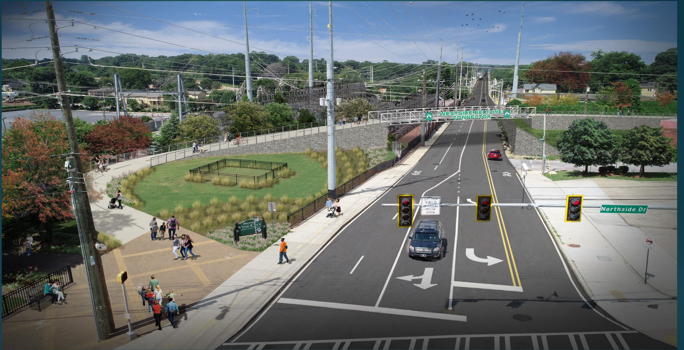
Boone Bridge - After
